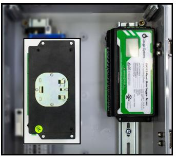
7) Attach the eGauge using the eGauge DIN rail mounting kit. There are many ways to install this kit - the image to the left shows a "flat" mount. The right angle bracket can be used for a vertical installation.
