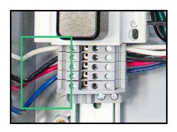
11) Wire the power distribution block to the breakers or fuse block of the distribution panel being measured. If using a grounded receptacle, be sure to connect the ground wire to the correct terminal block
