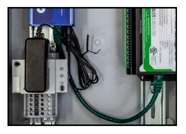
8) Connect the power adapter for the cell router (or other equipment) to the 120VAC receptacle and the Ethernet cable to the eGauge.
