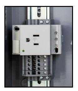
5) Add a terminal endstop to the side of the Phoenix 120VAC receptacle which is *not* in contact with the terminal blocks.
