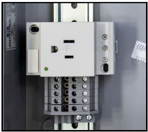
4) Connect the Phoenix 120VAC receptacle to the DIN rail, next to the terminal block *without* an end stop.
