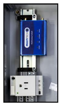
6) Attach the optional cell router or other equipment using DIN rail clips (eGauge provides DIN rail mounting kit and antenna extensions with the cell modem).
