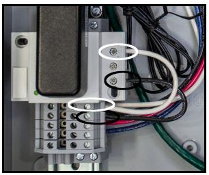
10) Cut lengths (approximately 7" long) from the white and black section of colored wire. Connect these to the Phoenix 120VAC receptacle (black to "L1" or "+", white to "N" or "-" and to the terminal blocks (match the colors to the existing wiring on the terminal block - black to black, white to white). If using a 3-prong grounded power adapter, connect a ground wire from an unused terminal block to the "PE" or "-" receptacle connection.
