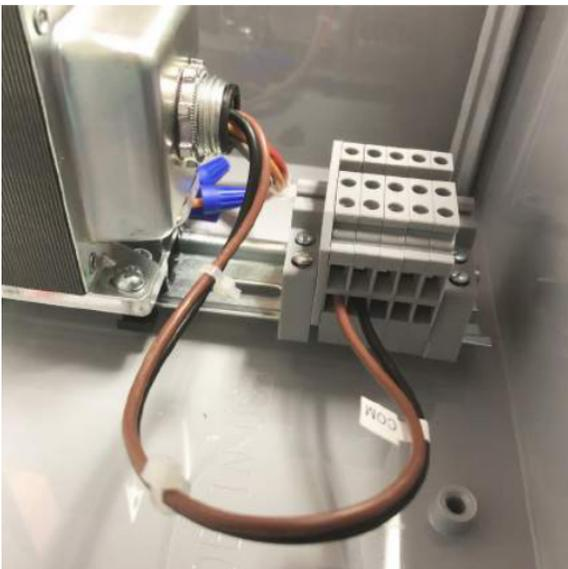
5) Insert the black and brown wires on the primary side of the transformer into the terminal block as shown in the photo. Use wire nuts or electrical tape to cover all exposed ends of unused wire on the primary side of the transformer.
