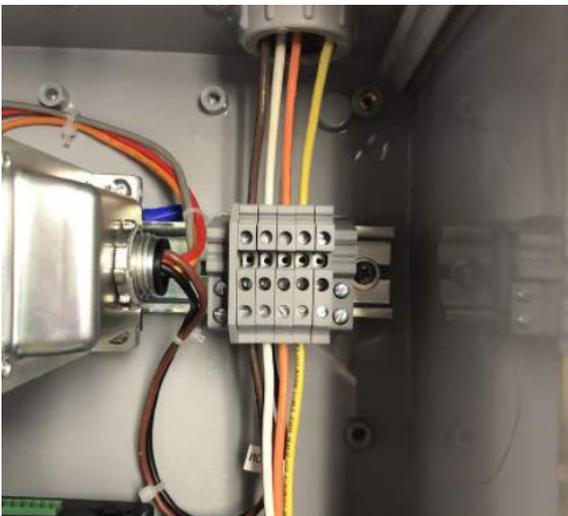
12) Wire the power distribution block to a breaker or fuse block of the distribution panel being measured.
