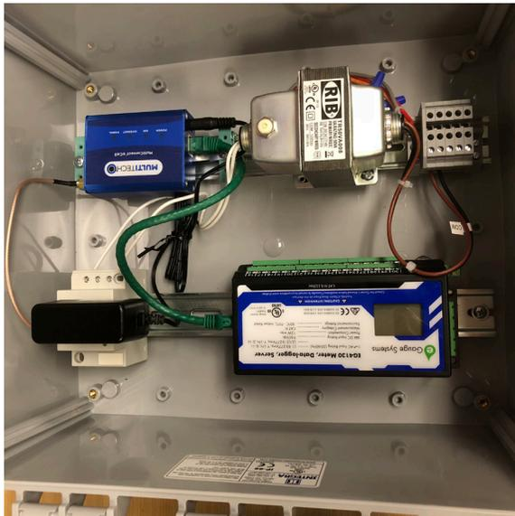
10) Connect the power adapter for the cell router or other accessory to the 120VAC receptacle and the Ethernet cable to the eGauge
