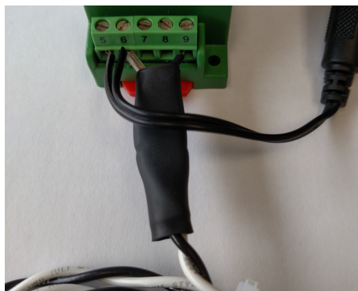
Figure 2: Completed CR5220 wiring
